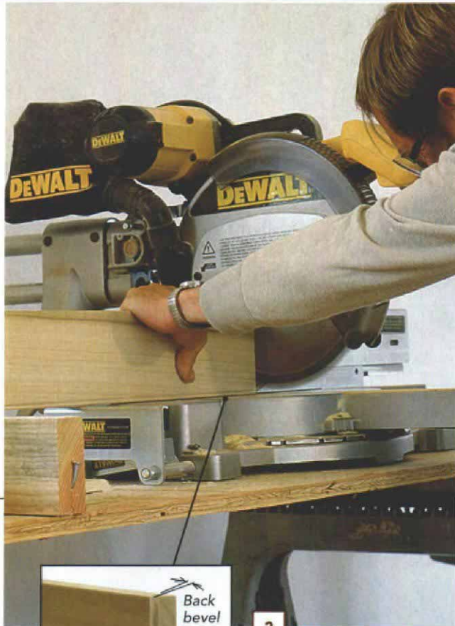
2 A flip and a plunge. The baseboard then is flipped upside down on edge, and the saw is plunged down the straight part of the profile at a slight back bevel.
