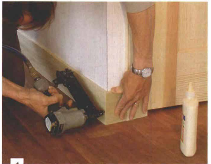
4 Glue and pin the joint.
